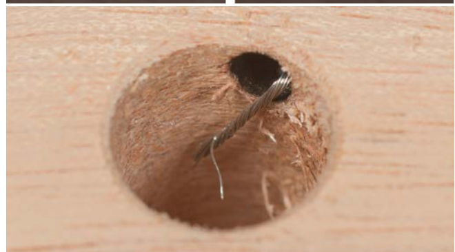
Ground wire in bushing hole
