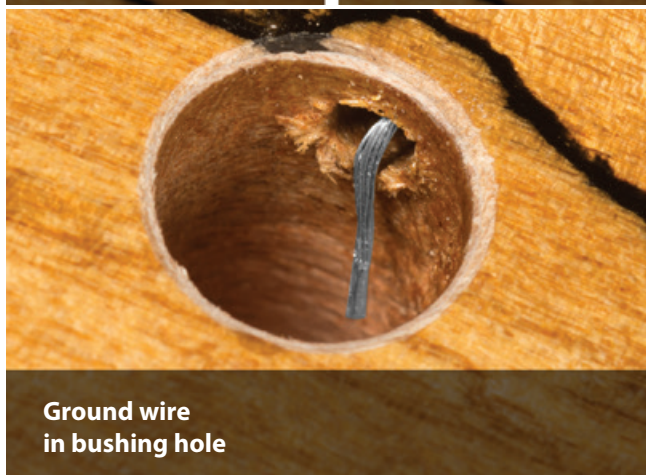
Bushing hole before chamfering
