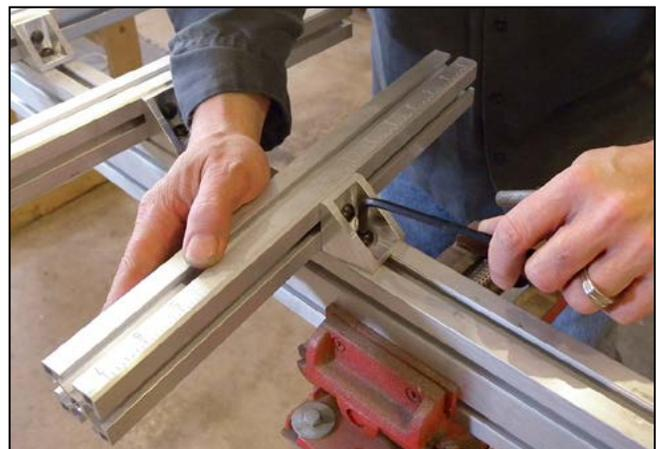
**1.** Install an angle support in each of the three crossbars. The T-shaped sliders fit the crossbars, and the square nuts are for mounting to the main beam. Two of the crossbars have etched centering scales, which should face upward.
