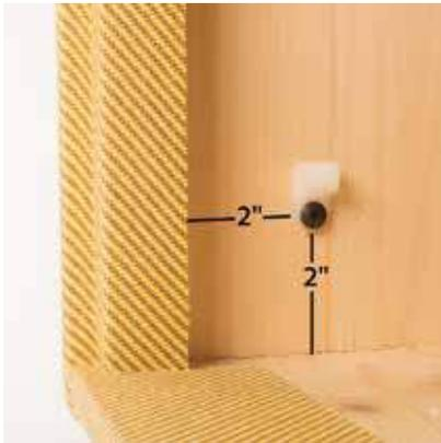
Don't drill through the cabinet! Use a piece of masking tape on your drill bit to mark the depth, or use a StewMac Depth-stop Drill Bit (item #1712).
